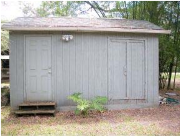
Large Storage Shed w/Electric
