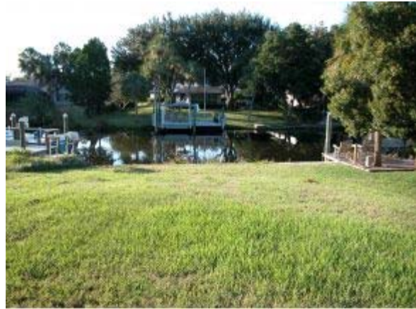
Ready with Fill and Seawall
