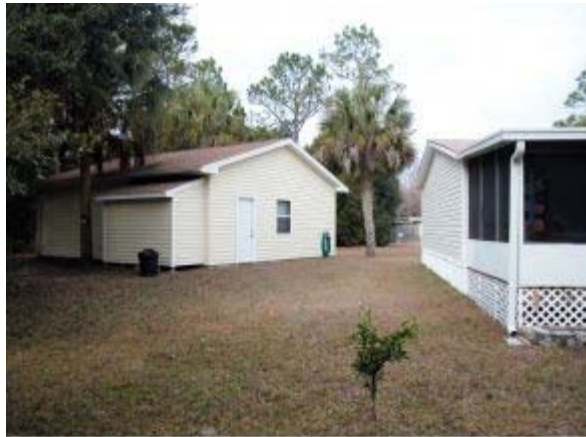
Garage with Bump-out
