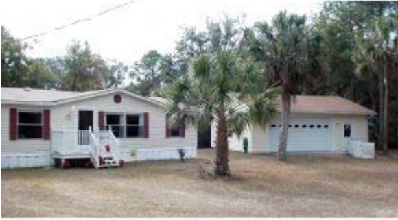
Perfect Condition - New Roof
