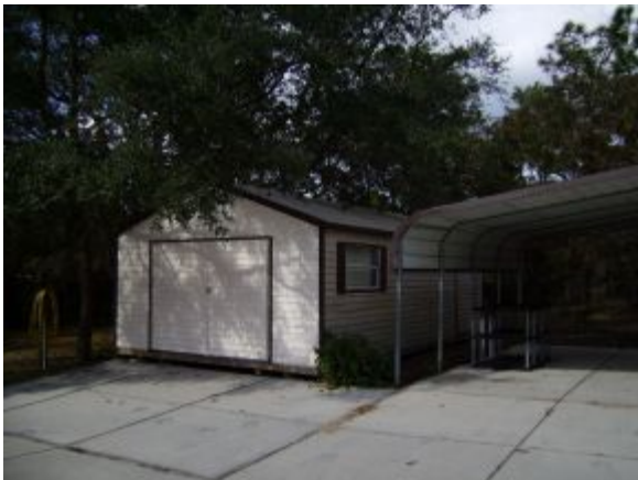
Workshop and Carport too!
