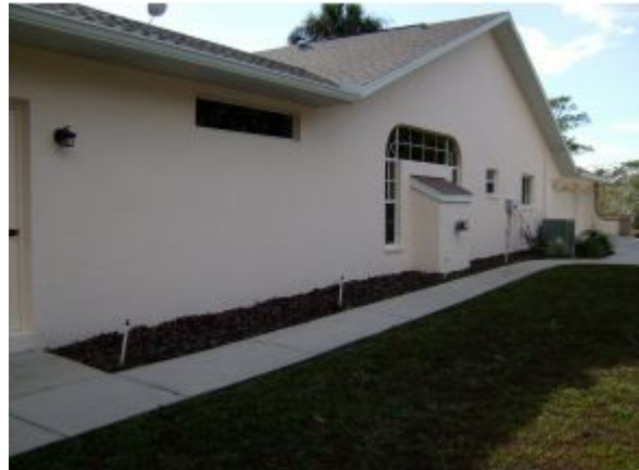
3 Car attached Garage
